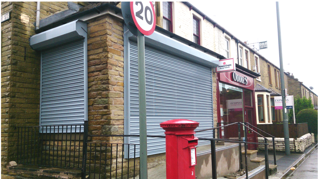
existing security shutters
